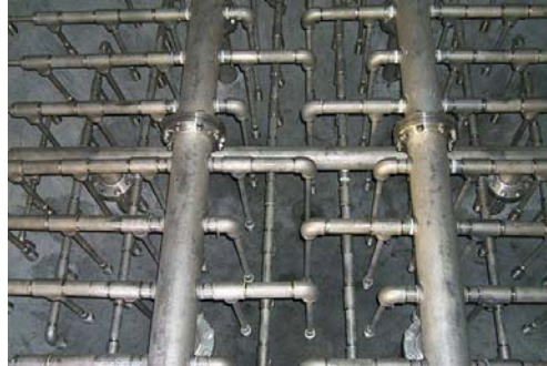
CUSTOM DROP LATERAL UNDERDRAIN SYSTEM
